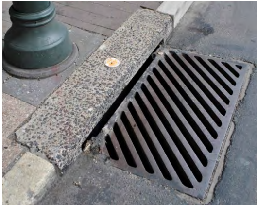
Storm drain network
