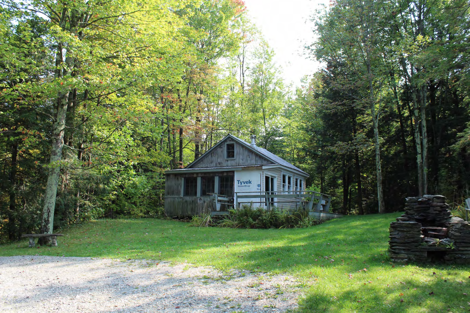
BEFORE: Small residence with roof & driveway runoff
