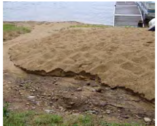
Deep rill formed after sediments and sand are washed into the lake leaving heavier stones behind.
